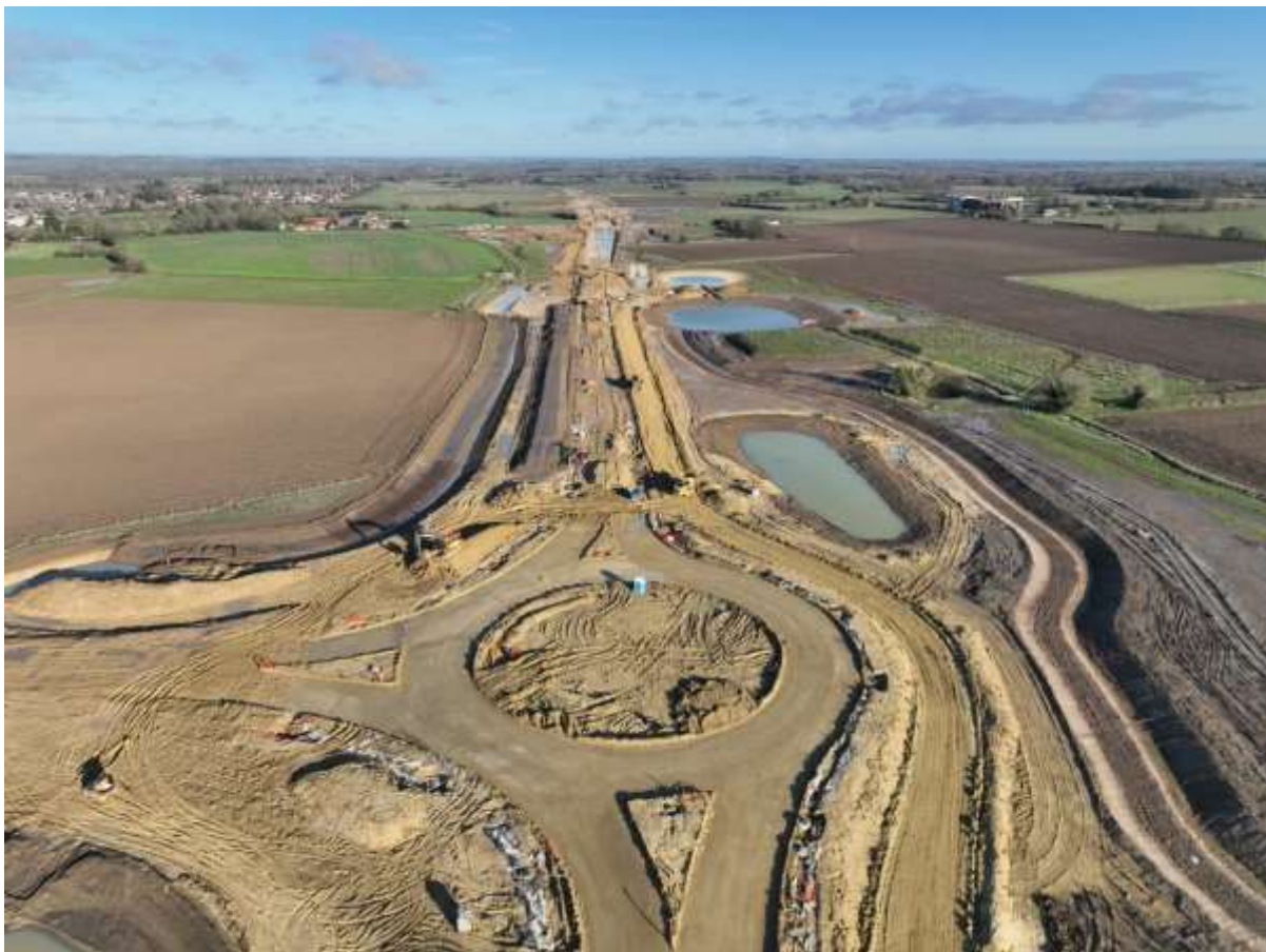
Figure 12 - Construction of the new roundabout junction at Church Lane, for the Long Stratton Bypass
