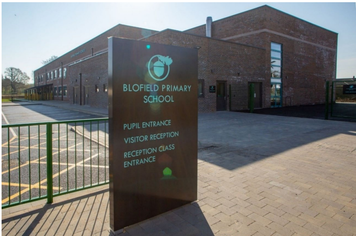
Figure 19 - Blofield Primary School.
